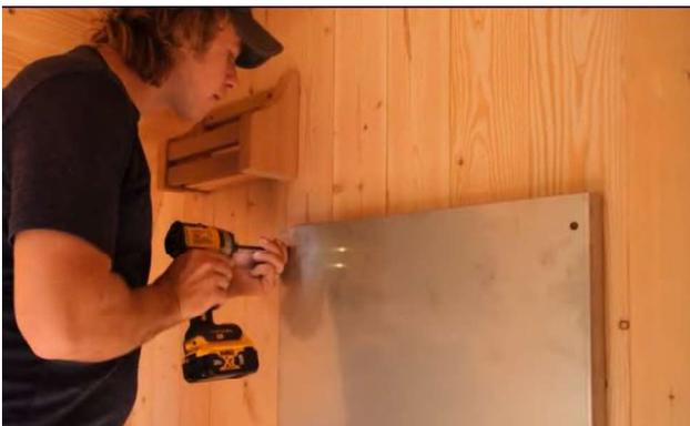
Place the rear wall heat shield and secure with 6 - 1 ½" (38mm) screws through the drilled holes.
