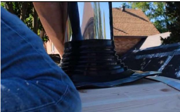
On the top of the sauna, pull the boot over the pipe, mark the outline of the boot.
