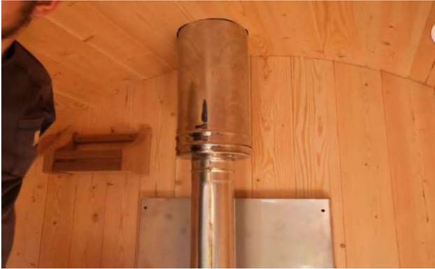
Place the first thick insulated chimney pipe on top of the first pipe and put it through the hole in the roof.
