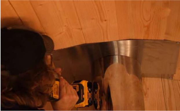
Install the 2 halves of the thin metal sheeting around the chimney on the inside to cover the hole.
